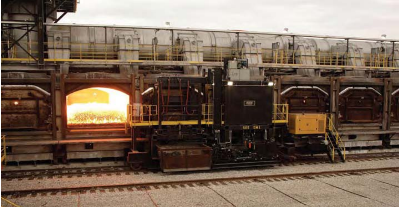
Fig. 20 Coke transfer car equipped with AP bearings
